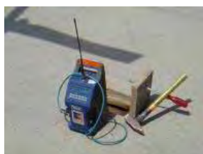
(Fig 4 Leakage detection)
