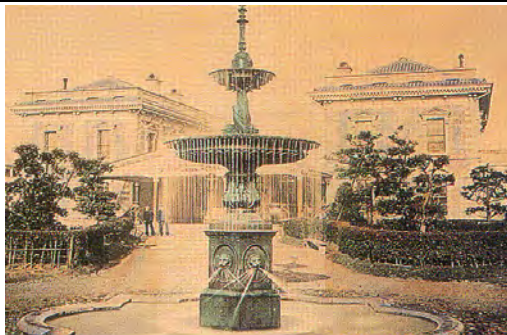
Y17 Public fountain in front of station
