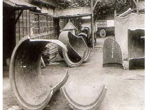
T18 Damages by earthquake in 1923
