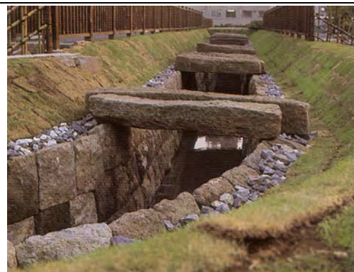
T29-2 Restored stone aqueduct
