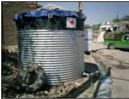
Temporary water supply tanks in Bam City
