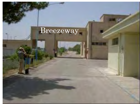
Picture 4-2-2 chemical House
