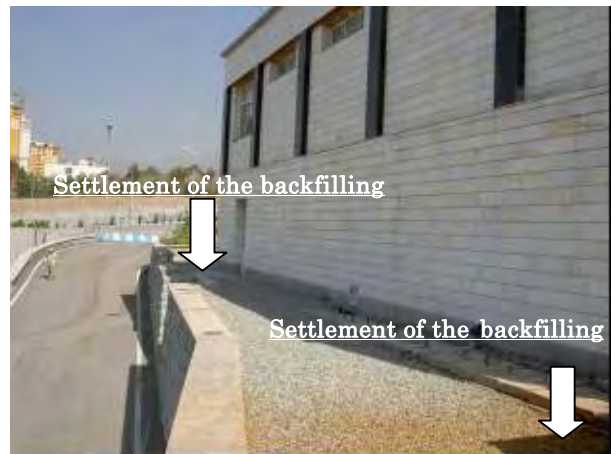
Picture 4-2-3 Chemical House
