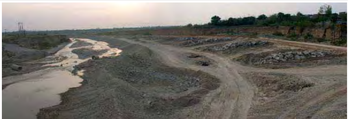
Before the 2005 Flood, Placement of Riprap Spur Dike
