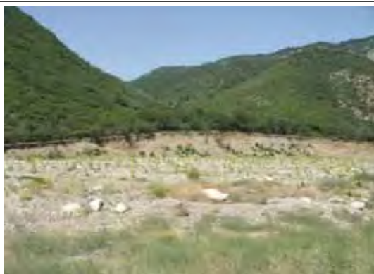
Serious Erosion along Riverbank and Fan End
