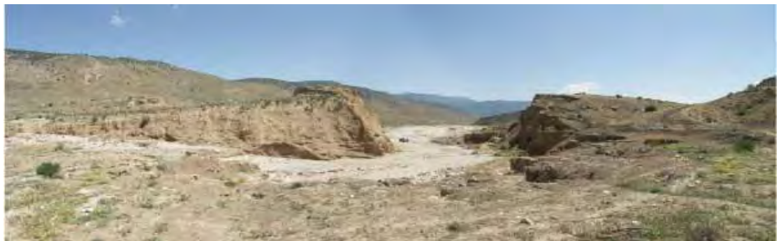
Breached Earth Dam viewing from Upper Point
