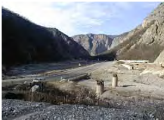
Destruction of Road connected to Mashhad
