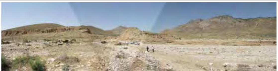
Breached Earth Dam viewing from Lower Point
