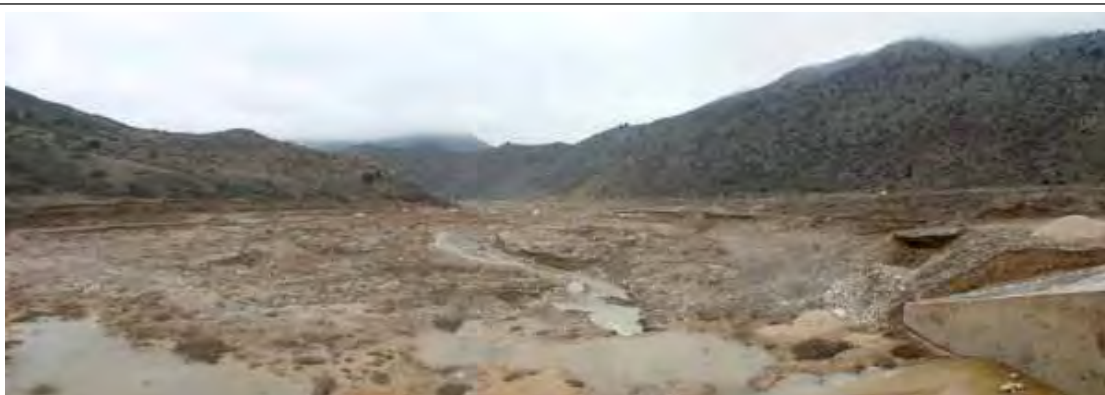
Downstream View of Dasht Bridge
