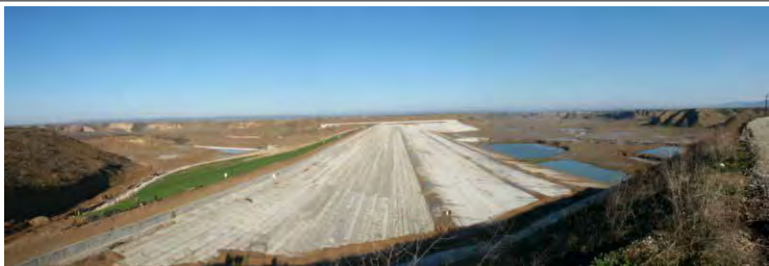
Golestan II Dam (under construction, December 2004)
