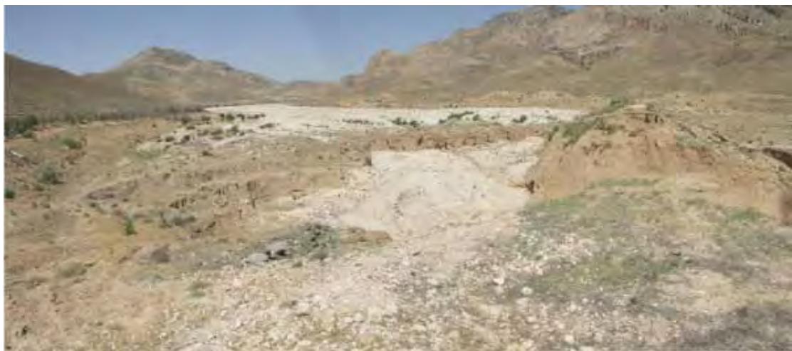
Stored and Eroded Sediment in the Basin of the Earth Dam
