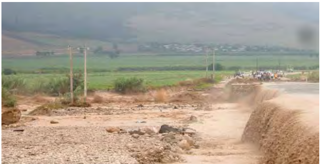
Overtopping the Gorgan-Mashhad Road
