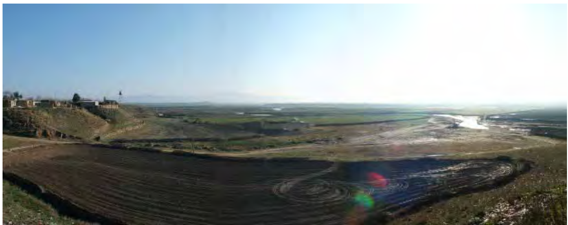
Upstream View of Lower Madarsoo from Right Bank, Khojehlar village (downstream of Kalaleh Bridge)
