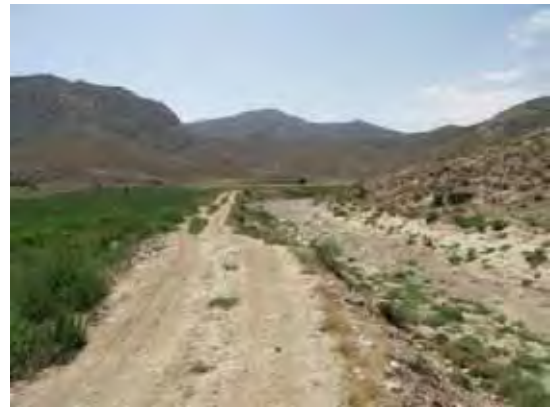
New Excavated Canal after the 2001 Flood
