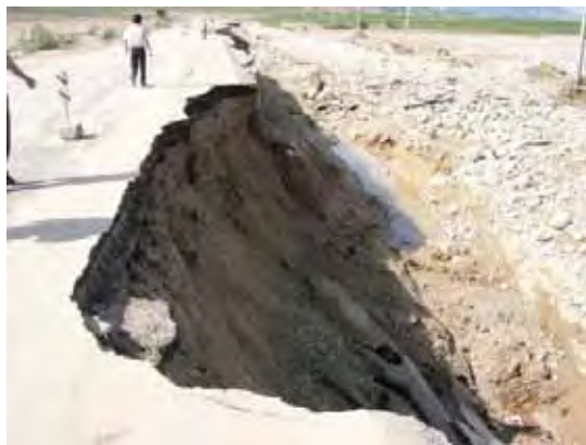
Damage on the road Embankment
