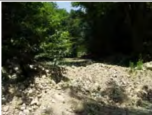
Debris Deposits near Tangra Entrance
