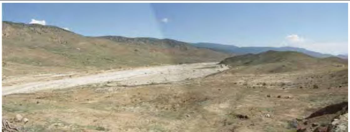
Downstream Stretch of Breached Earth Dam
