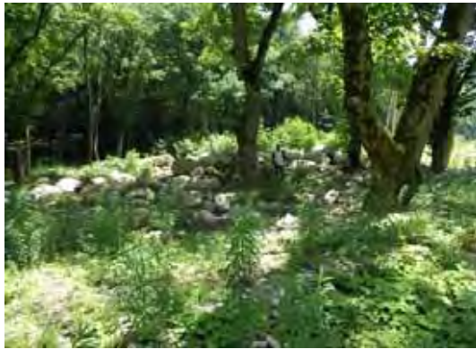
Debris Deposits near Tangra Entrance
