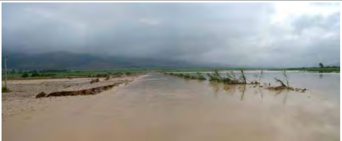
Flooding upstream of 14 Metry Bridge
