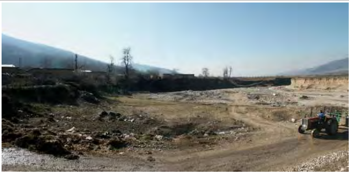
Loveh Bridge was washed out, and serious bank erosion occurred along the downstream bend.
