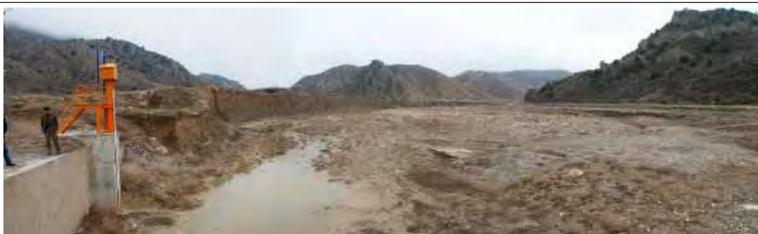
Upstream View of Dasht Bridge
