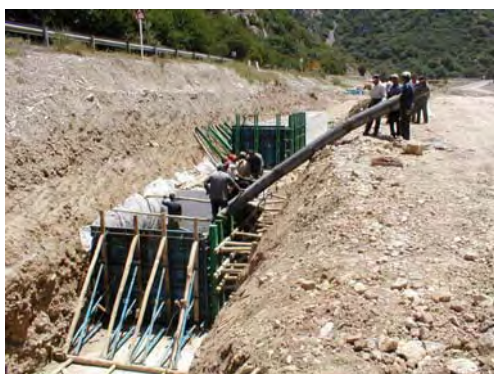
Photo 2.12 On-going Retaining Wall Work downstream of Golestan Tunnel (1) (Concrete Wall)
