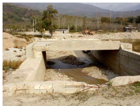
Photo 2.5 Existing Bridge No.7
