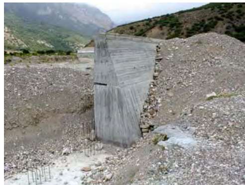
Photo 2.11 Completed Retaining Wall Work upstream of Golestan Tunnel (2)
