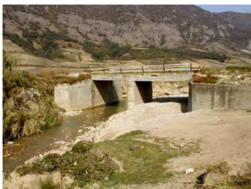
Photo 2.4 Existing Bridge No. 6
