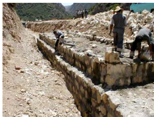
Photo 2.13 On-going Retaining Wall Work downstream of Golestan Tunnel (2) (Limestone Masonry)
