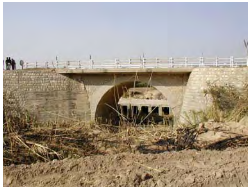
Photo 2.2 14 Metry Bridge (Existing Bridge No.3)
