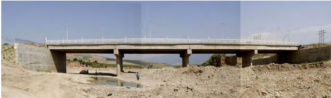
Photo 3.1 Reconstructed Kalaleh Bridge (L=84M) (No.1)
