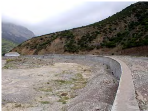
Photo 2.10 Completed Retaining Wall Work upstream of Golestan Tunnel (1)
