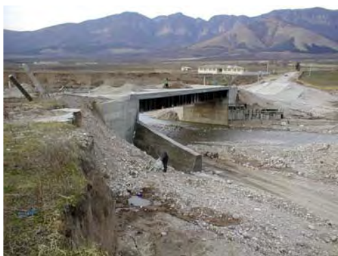
Photo 2.3 Reconstructed Loveh Bridge (No. 5)
