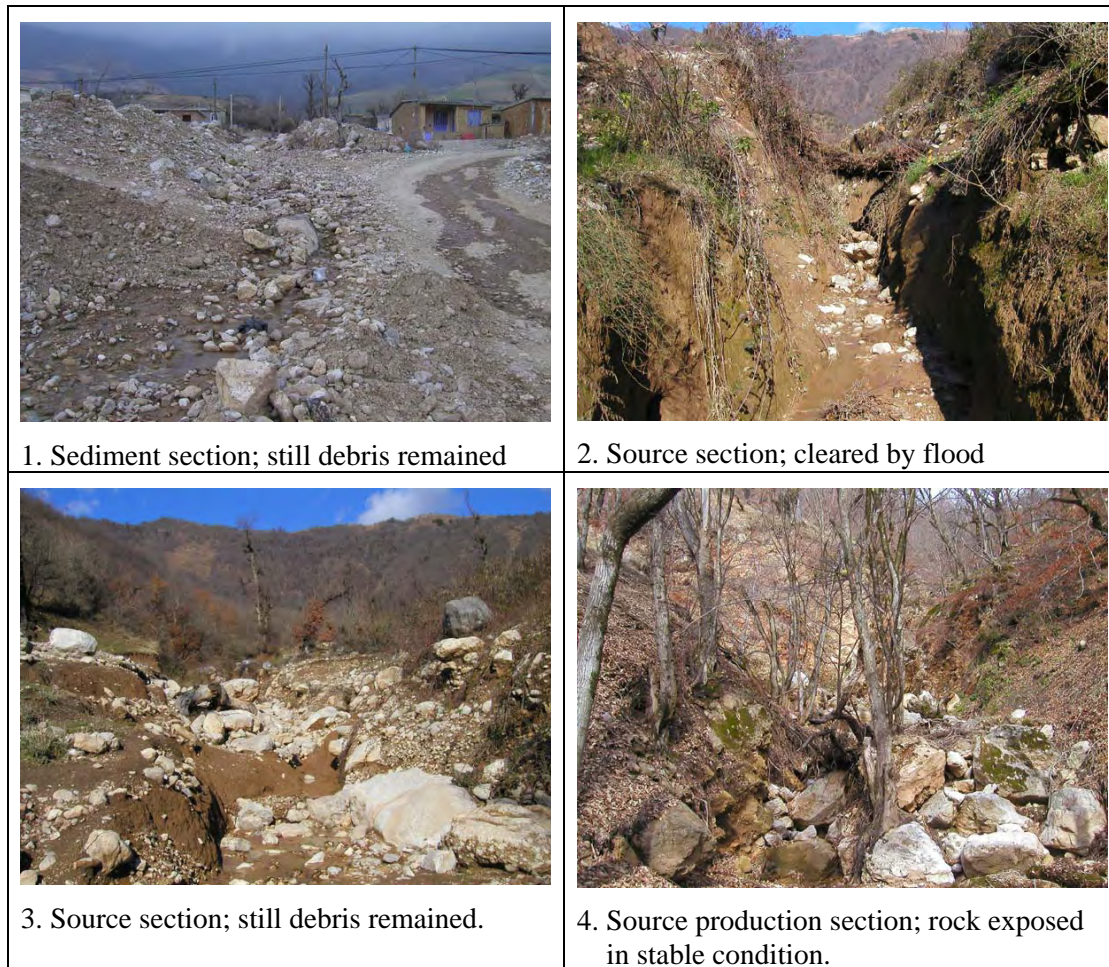
Figure 4.6 Debris Condition in T4 Valley
