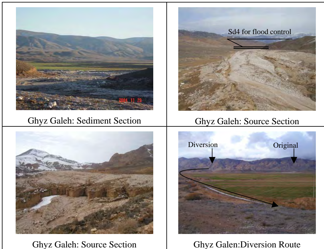
Figure 4.15 Debris Condition in the Ghyz Galeh
