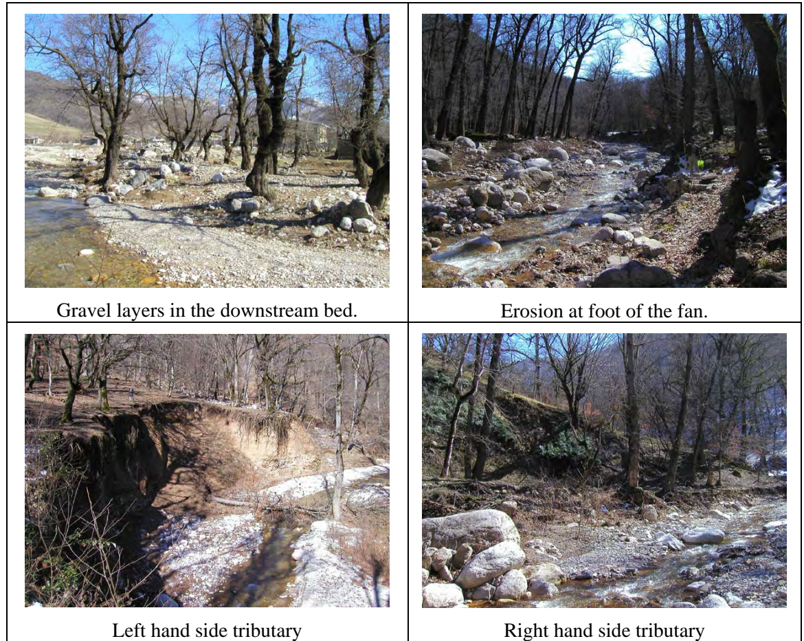
Figure 4.3 Debris Condition of T1 Valley
