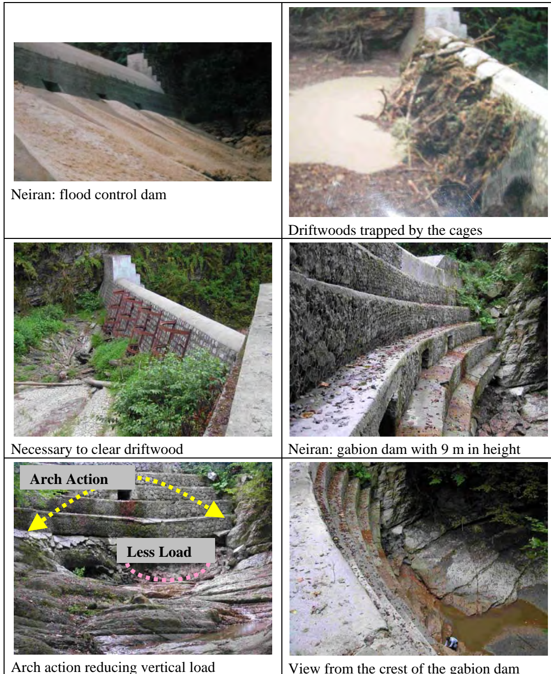
Figure 2.3 Neiran River Basin in Mazandaran
