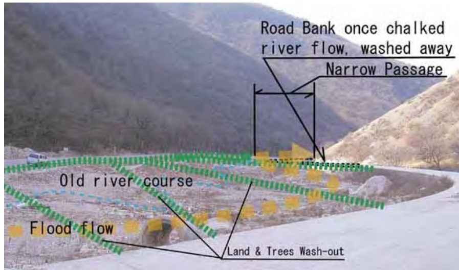
Figure 1.8 Road Bank Washed away by the Dammed-up Floodwater in 2001
