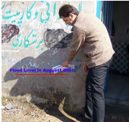
Fig. 6.3 Engineering Field Adjustment in Gharavol Haji Tajy village
