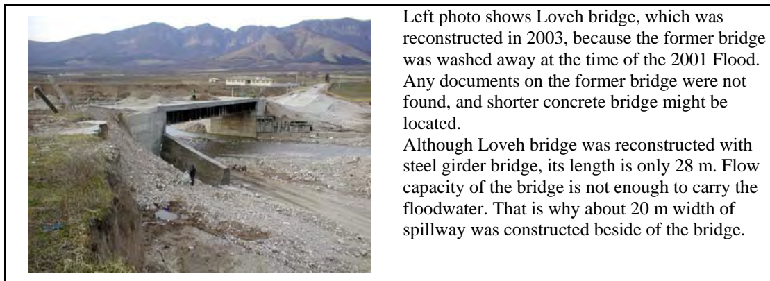
Fig. 2.100 Reconstructed Loveh Bridge (Bridge No. 5)
