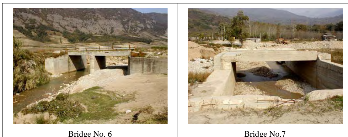
Fig. 2.101 Existing Bridges No. 6 and No. 7
