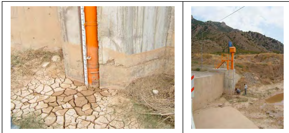
Fig. 2.111 Dasht Water Level Gauging Station
