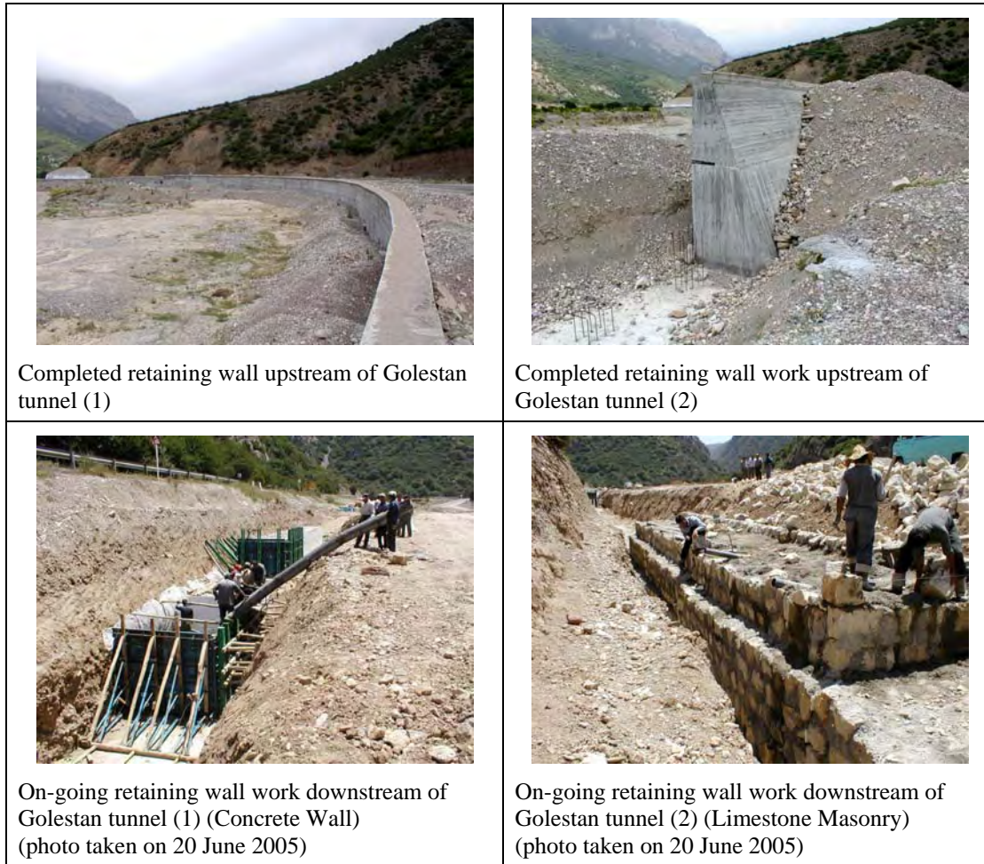
Fig. 2.104 On-going Road Construction Work in the Golestan Forest
