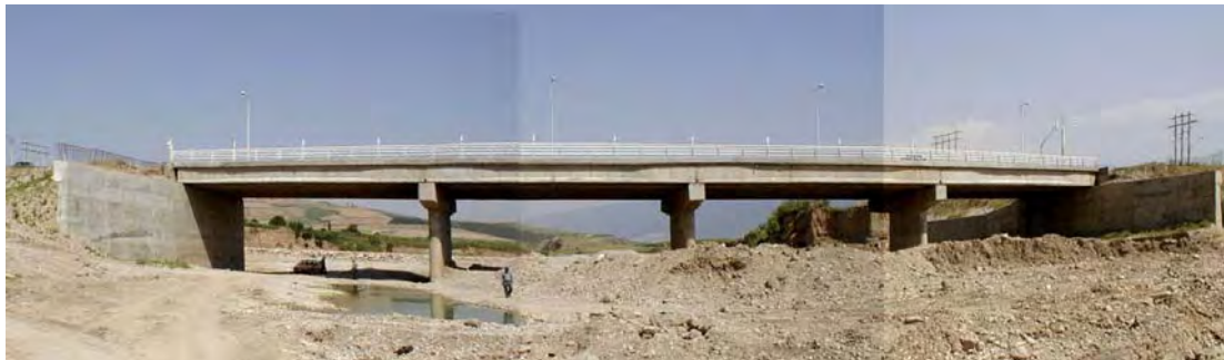
Fig. 2.97 Reconstructed Kalaleh Bridge (L=84 m) (Bridge No.1)
