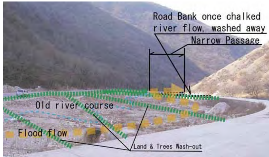
Fig. 2.8 Road Bank Once Chalked the River Flow and Washed Away by the Flood
