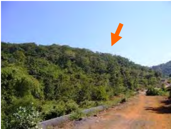
Photo M113.1.1 Outer appearance of Sirvoi MBR.
