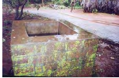
Storage tank outside the house. Habitants totally dependent on tanker water.
