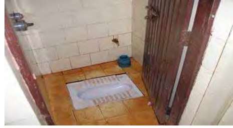
Example of Indian water close let type toilet with flushing system in sulabh toilet
