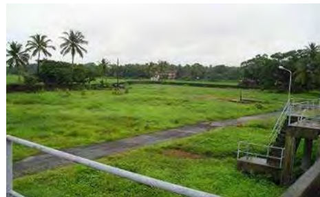
Around Margao Sewerage Treatment Plant
