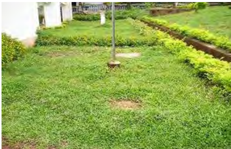
Septic tank covered with grass in a hotel
