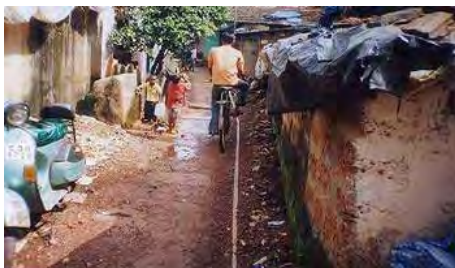
Metered stand post / metered water connection outside house shared by 2 to 3 houses in Monte Hill , Margao
