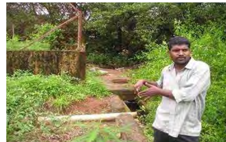
Discharge point of Panaji Commercial STP
