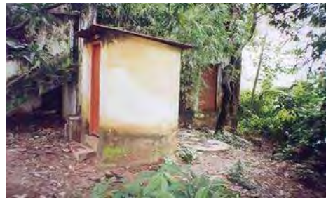
Open well and toilet very closely placed
