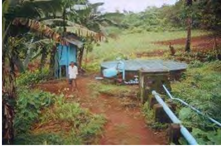
Regional water supply scheme source, open well
