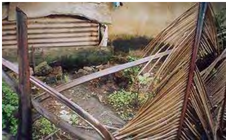
House wastewater discharged into open ground
