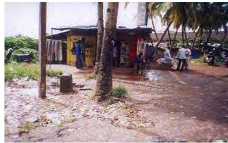
Public stand post leaking water
