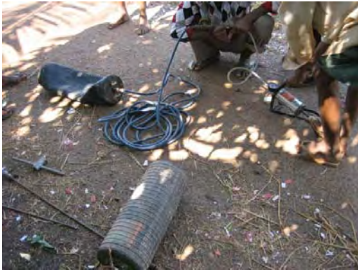
Photo 32.7 Balloons to close sewer
