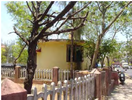
Photo 32.1 Outside View of P/S-3
