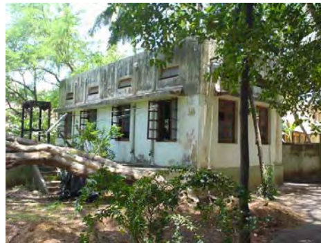
Photo 32.2 Outside View of P/S-5
