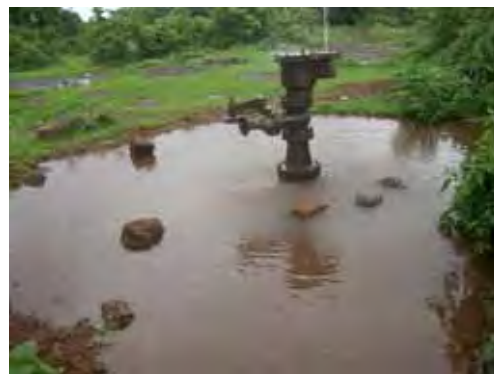
Photo 31.7 Leakage from Air Valve along the Transmission Main
