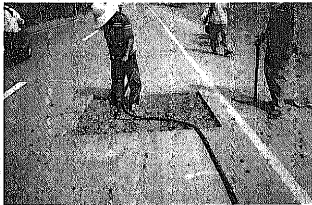
Hacking asphalt concrete
