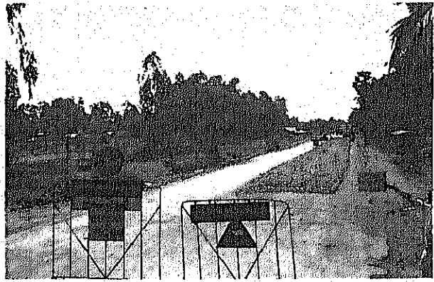
Repairing by RCC (1999)
