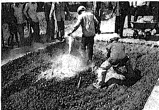
Placing new base course and stabilizing by cement t = 20\text{cm}
