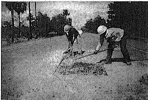
Placing new base course and stabilizing by cement t = 15\text{cm}
