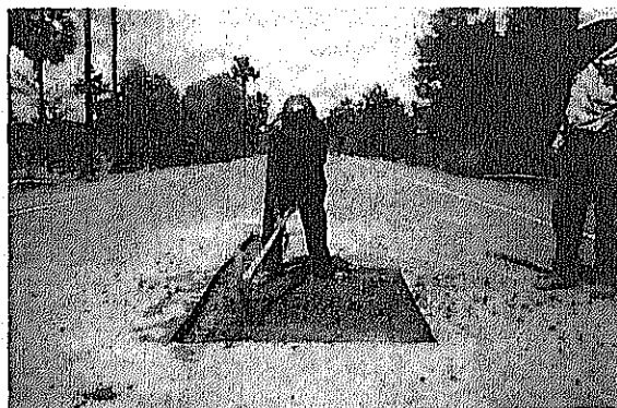
Removing base course
