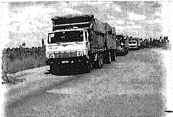
Damaged Road National Road No.5
