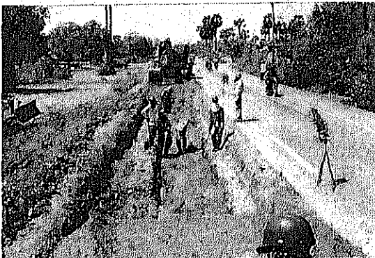
Replacing by sand t = 30\text{cm}
