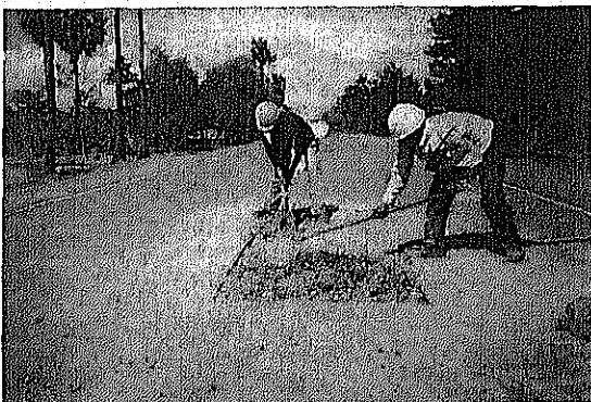
Placing new base course and stabilizing by cement t = 20\text{cm}
