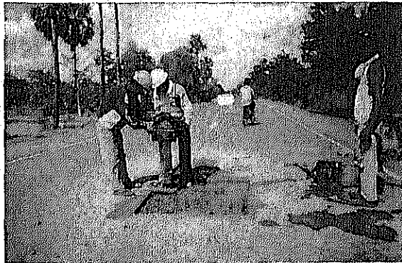
Compaction of new base course
