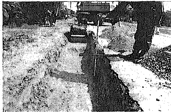
Replacing by sand t = 30\text{cm}
