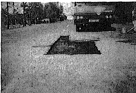
Spreading prime coat
