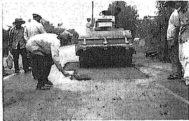
Compaction by Roller 7ton
