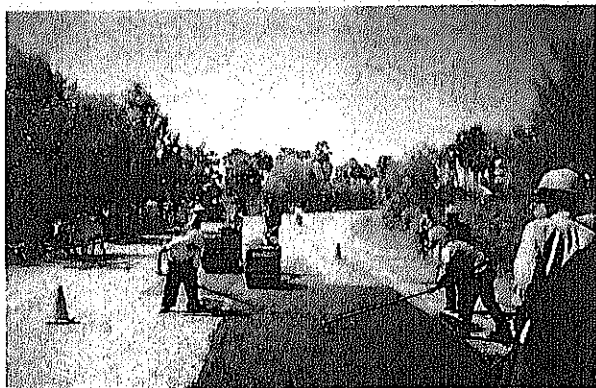
Compaction by Roller 1.0t
