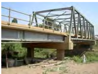
Steel Girder + Truss (NR.5)
