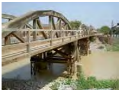
Concrete Truss Bridge (NR.31)
