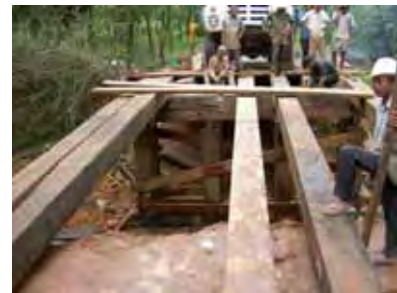
Timber Bridge under Repair (NR.78)
