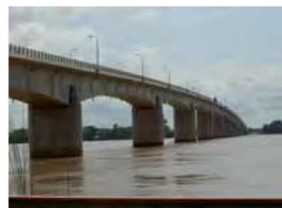
Kizuna Bridge (PC Box)(NR.7)
