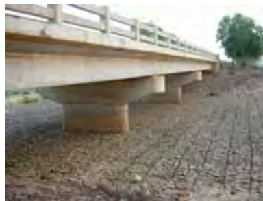
Concrete Bridge (NR.6)
