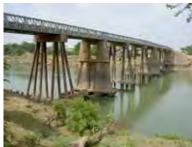
Bailey Bridge (NR.11)
