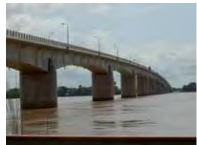
Kizuna Bridge (PC Box)(NR.7)
