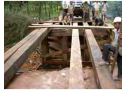
Timber Bridge (NR.78)
