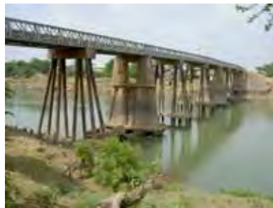
Bailey Bridge (NR.11)
