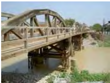
Concrete Truss Bridge (NR.31)
