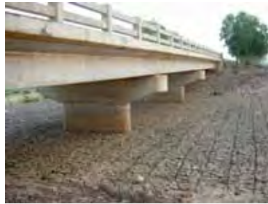
Concrete Bridge (NR.6)
