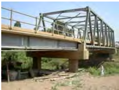
Steel Girder + Truss (NR.5)
