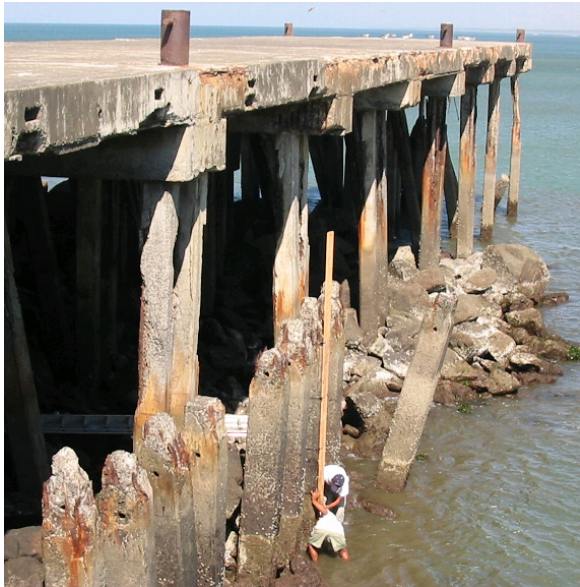
Photo 8-9 Installation of Tide Scale
