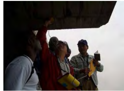
Deterioration Survey (Port Saco Mar)
