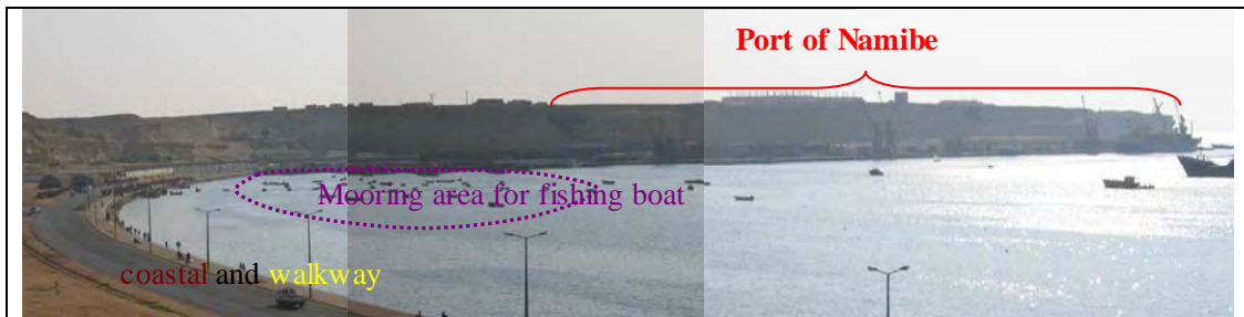
Photo 7-14 Panoramic view of Port of Namibe
