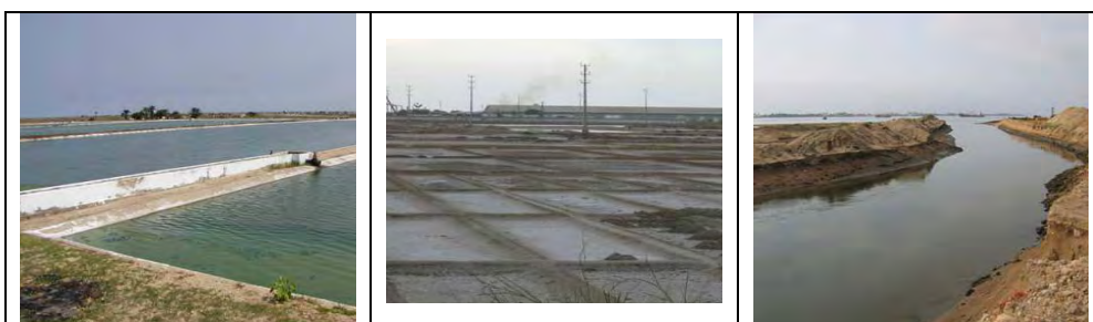
Photo 7-9 Sewerage facility, Salt pot and water channel to Lobito bay
