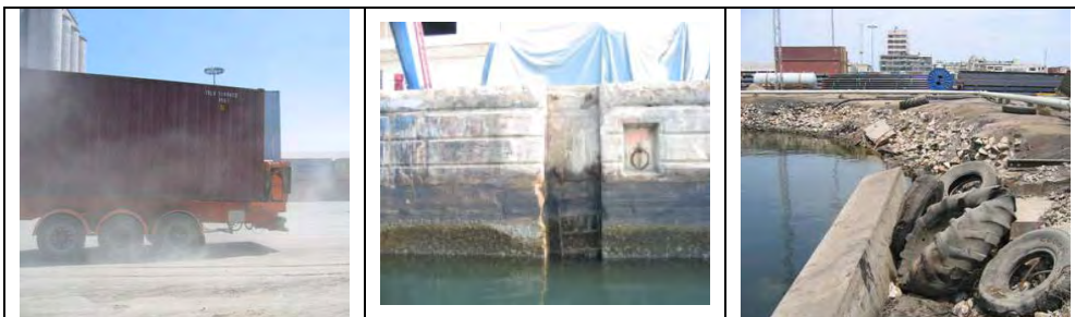
Photo 7-13 Dust in unpaved yard, Damaged safety rudder, and South quay
