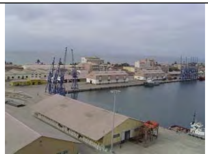
Warehouse closed to the quay front
