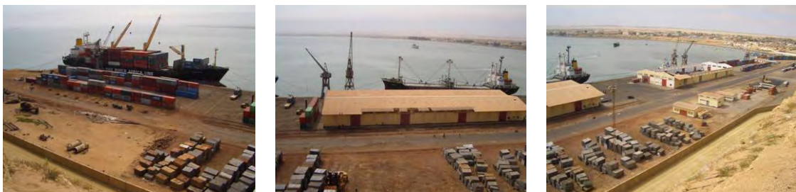
Photo 5-18 Panoramic View of Port of Namibe (2005)
