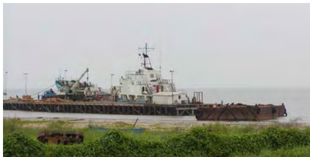
Photo 5-23 Port of Cabinda in May, 2005
