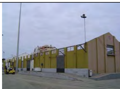
Repair of No. 10 warehouse in the north wharf
