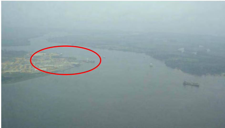
Photo 5-24 The Port of Soyo (in red circle)
