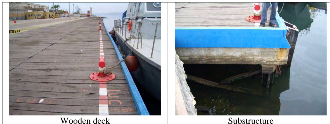
Photo 5-17 Present Status of the Cabotage Jetty
