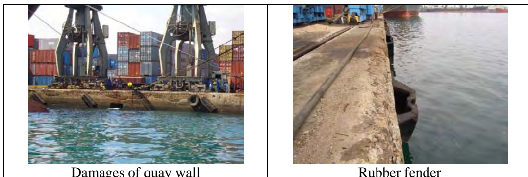
Photo 5-12 Conditions of Quay Wall and Rubber Fenders
