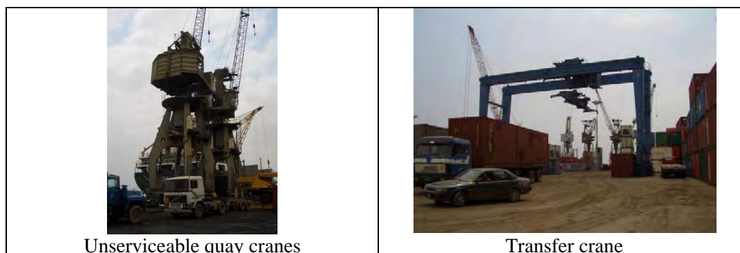
Photo 5-13 Cranes of the Container Terminal
