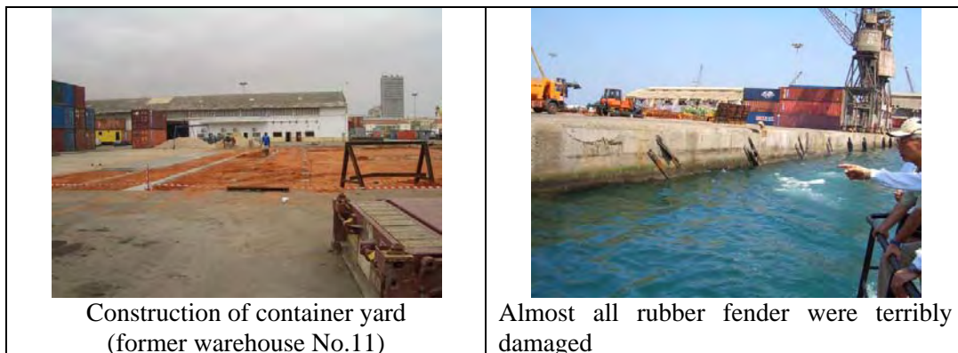
Photo 5-9 Conditions of South Side of the General Cargo Terminal
