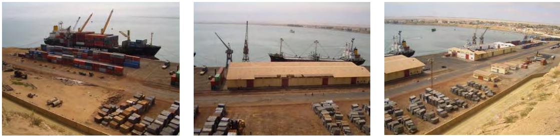
Photo 5-3 Panoramic View of Port of Namibe (2005)
