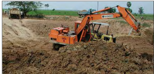
Backhoe excavation of the area of drying bed Casting concrete and checking finishing
