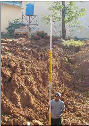
Check the excavation bottom level
