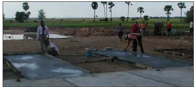
Backhoe excavation of the area of drying bed Casting concrete and checking finishing
