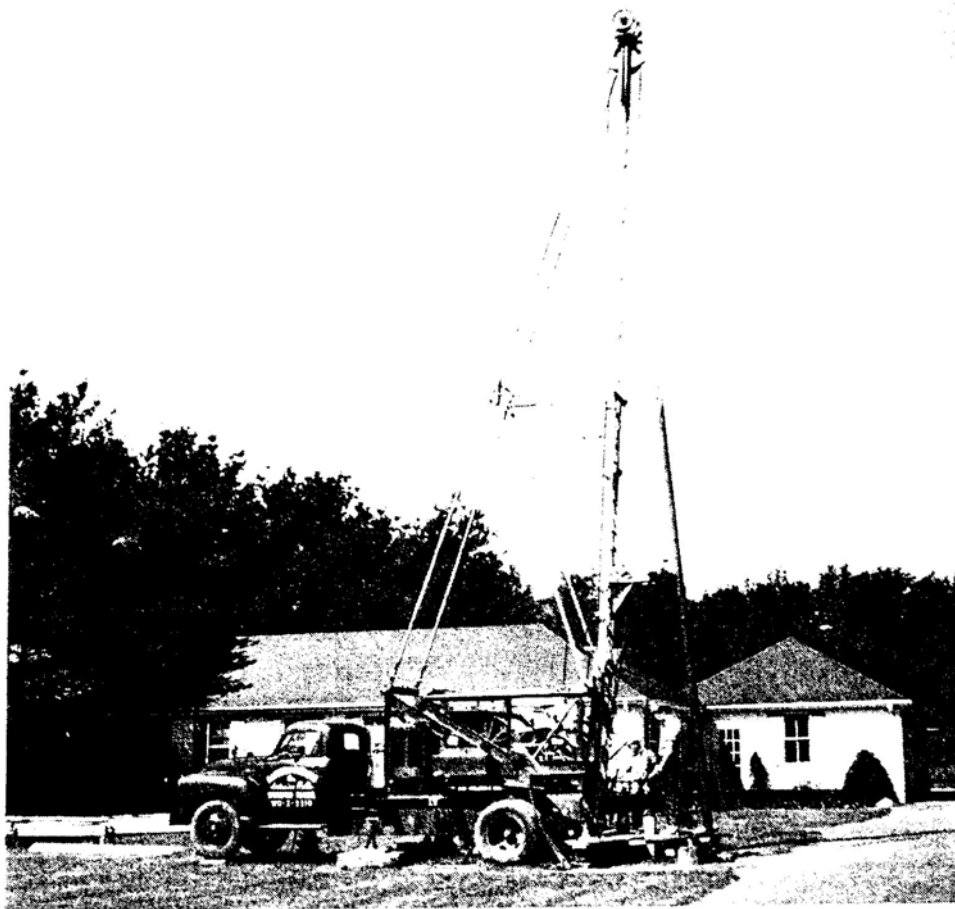
Figure 1.1-2: Cable Tool Rig in Operation
