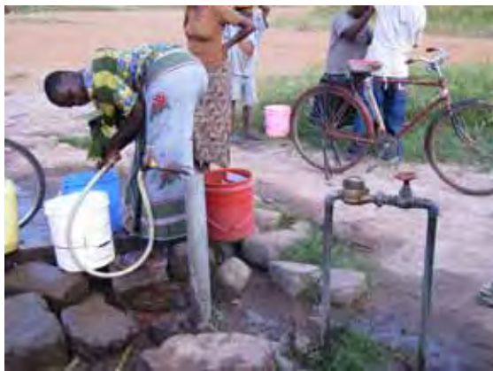
Communal Tap with Meter
