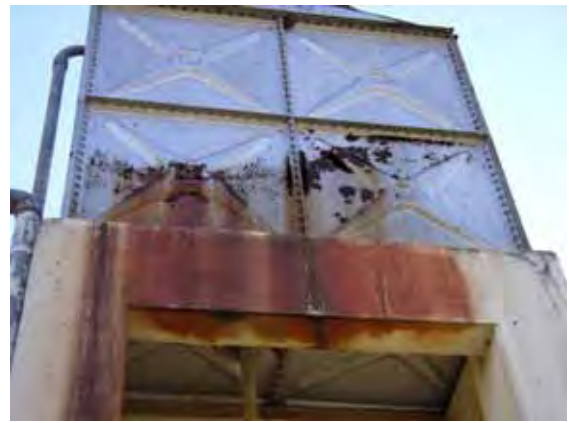
Corrosion of Water Tank
