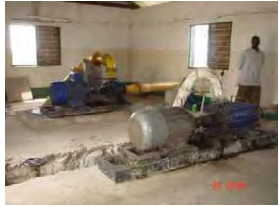
Breakdown of Pumping Machine
