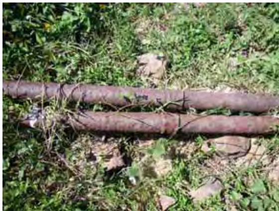
Deterioration of Pipes
