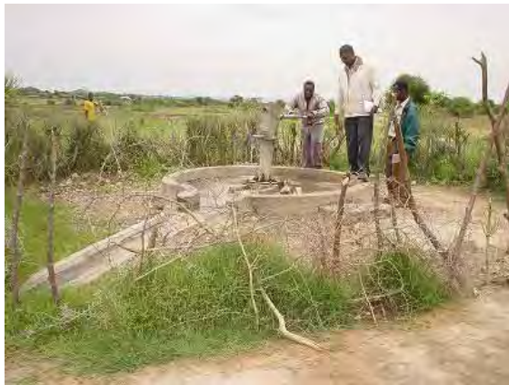
Hand Pump Facility with Platform
