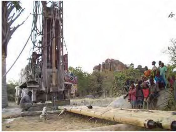
Setting of Drilling Rig
