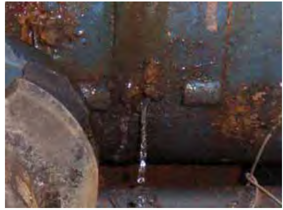
Leakage in Pumping Machine
