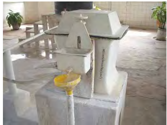
Water Quality Control (Pouring Chlorine)
