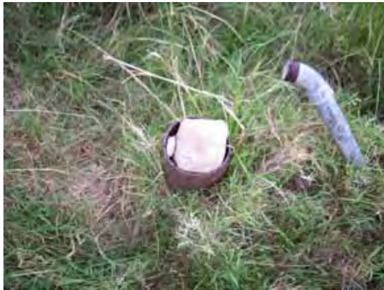
Abandoned Water Pipe
