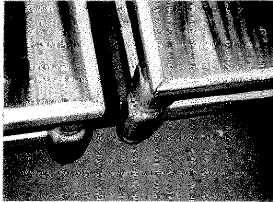
Photograph 1 Miter joints with chinks
