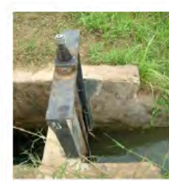
Turn out gate #48
