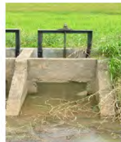
Turn out gate #36
