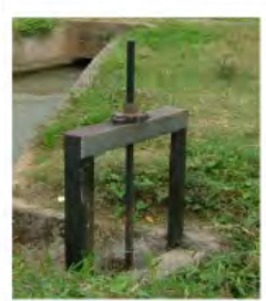
Turn out gate #54
