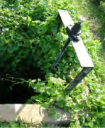
Turn out gate #45
