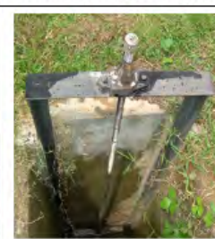
Turn out gate #62
