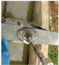
Turn out gate #40
