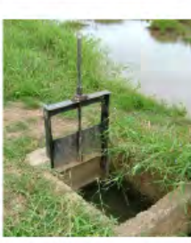
Turn out gate #57
