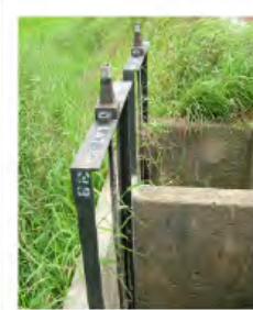
Turn out gate #38
