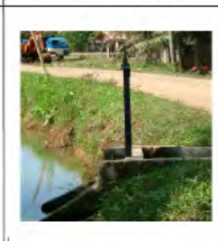
Turn out gate #64
