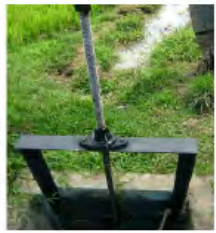
Turn out gate #26
