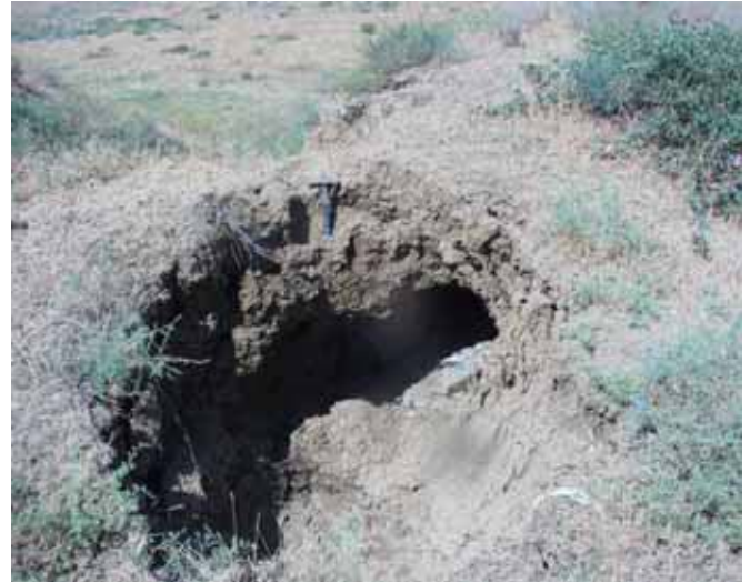
Piping hole, 1 meter diameter which was admitted in the clay soil of hard weathered sedimentary rock
