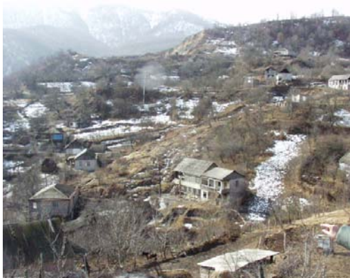
Figure 9.5 General View of H block of Gosh Village Landslide
