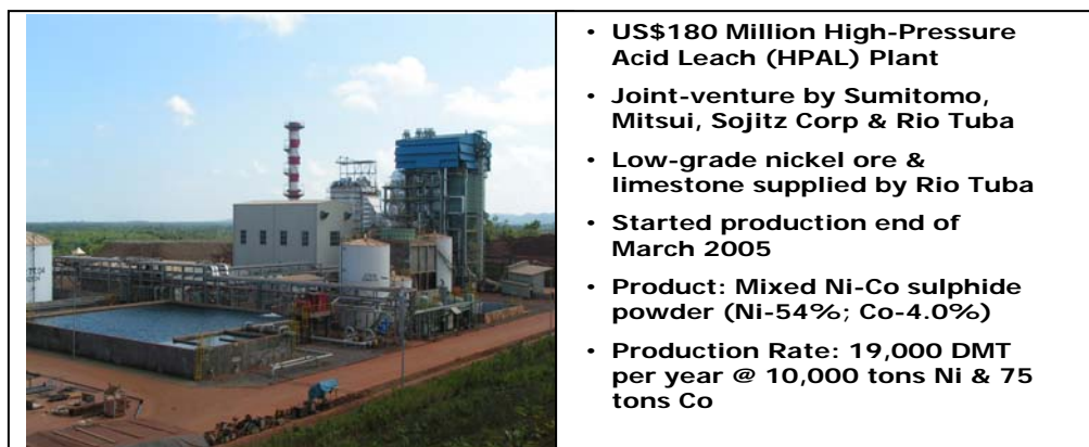
Figure 4. Profile of the Palawan Nickel Project of the Coral Bay Nickel Corporation
