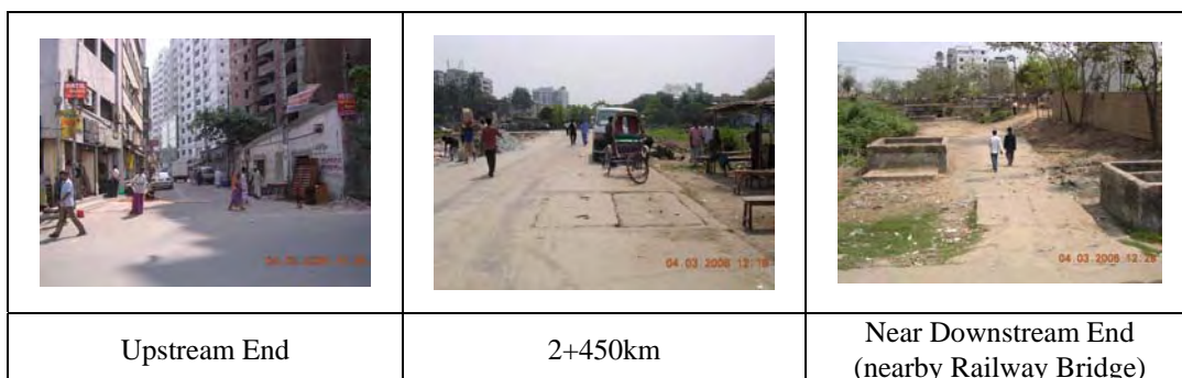
Photo 2.3 Present State of the Box Culvert in Segunbagicha Channel
