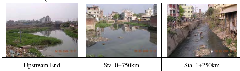
Photo 2.4 Present State of the Open Channel Stretch of Segunbagicha Channel
