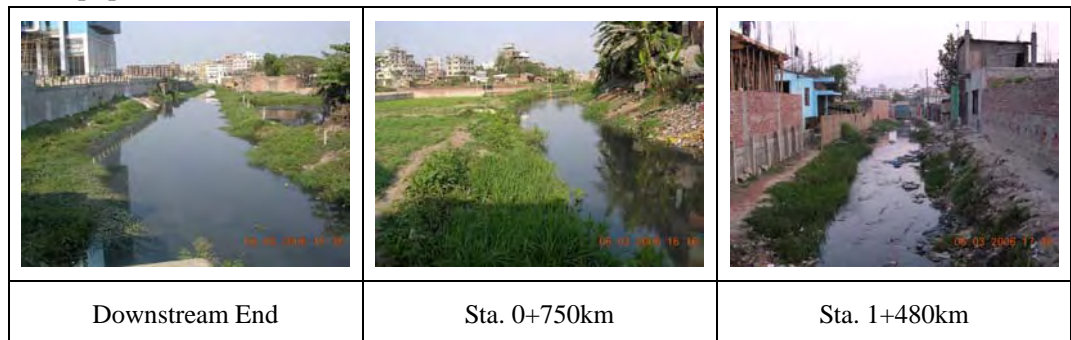
Photo 2.6 Present State of the Mirpur Channel
