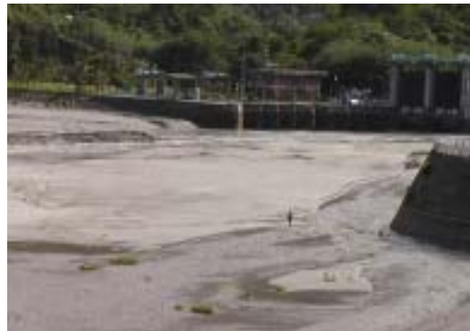
View from the Upper Stream of Bakaru Reservoir
