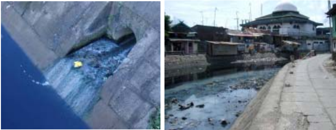
Photo 2.1 Graywater Flowing into Public Water Body without Treatment
