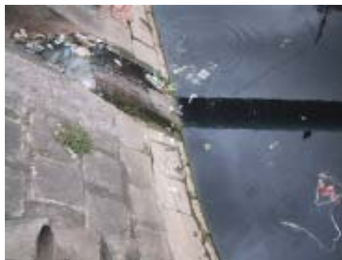
(Solid waste flowing into main canal)
