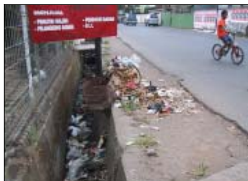
Stuck drainage where solid waste is dumped
