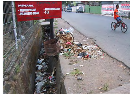
Stuck drainage where solid waste is dumped
