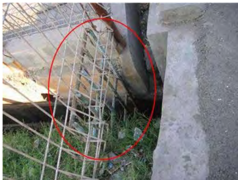
Fence in a drainage (center)
