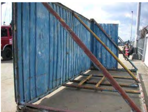
Mobile fence made of container (The inner bent part is a door.)
