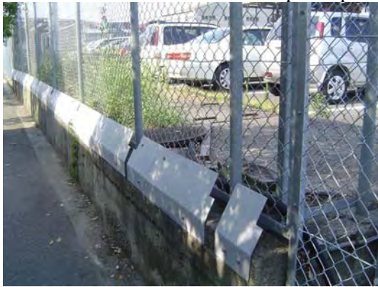
Photo 15-2-3-12 Sample Improvement of Concrete Foundation
