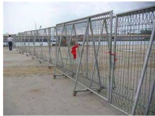
Mobile fences are in use as a partition between international vessel and domestic vessel.
