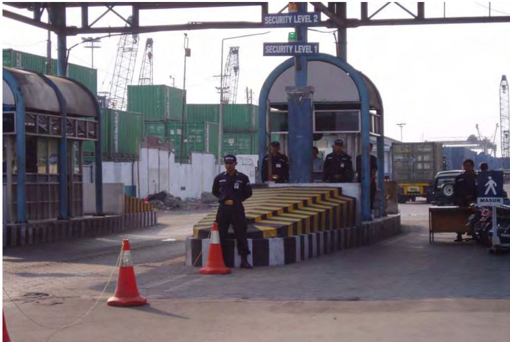
Access Control Gate (2)
