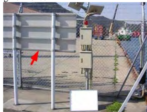
Independent sign board inside the restricted area (Red arrow shows the back side of sign board.)
