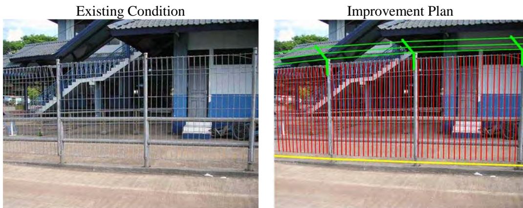
Photo 15-2-3-1 Improvement Plan of Grid Fence
