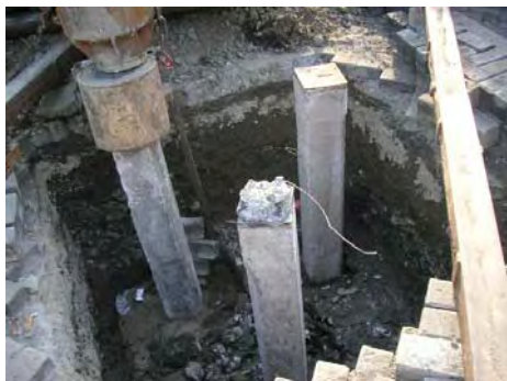
Camera pole base pile
