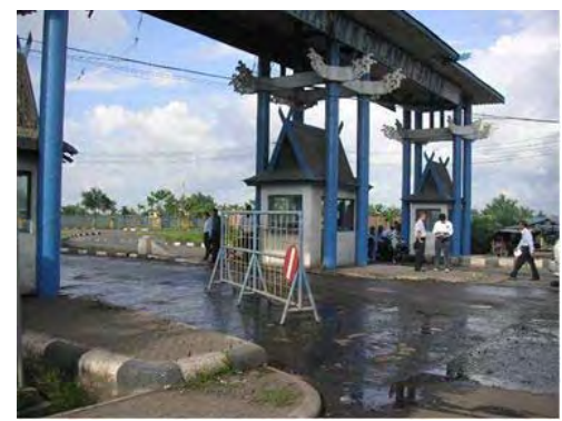
Mobile fence is used for the fence to prohibit vehicles to pass through.
