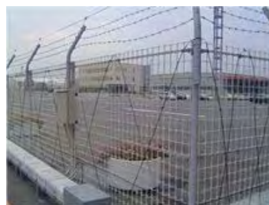
Outward angled top guard added on top of the existing fencing
