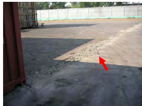
Buried piping backfill section
