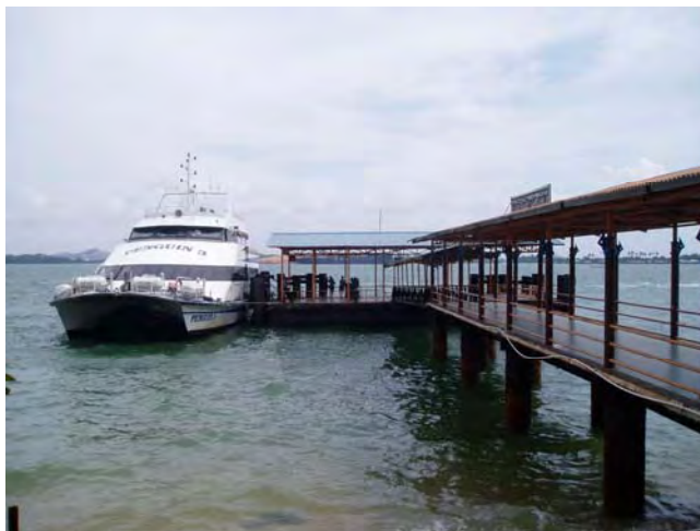
Photo 8-4-4-1 Pontoon for International Passenger Ship at Sekupang Terminal
