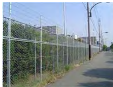
Mesh fence and upright top guard added on top of the existing fencing
