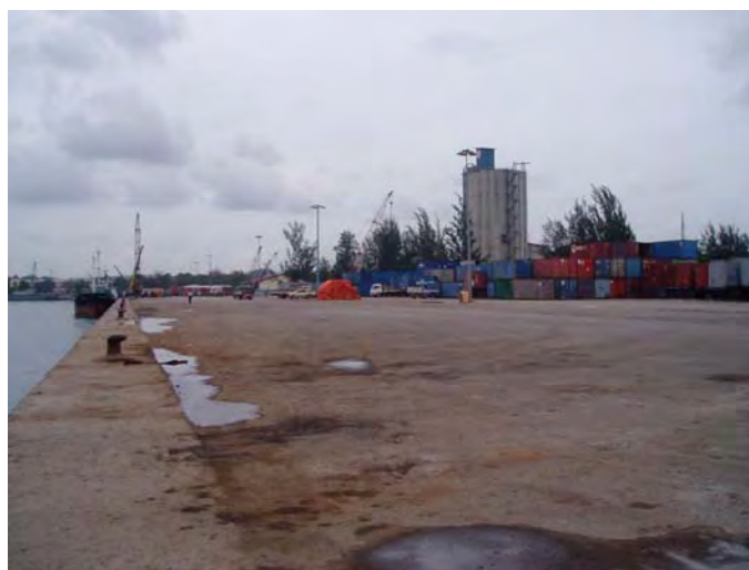
Photo 8-4-2-1 International Berth at Batu Ampar Port
