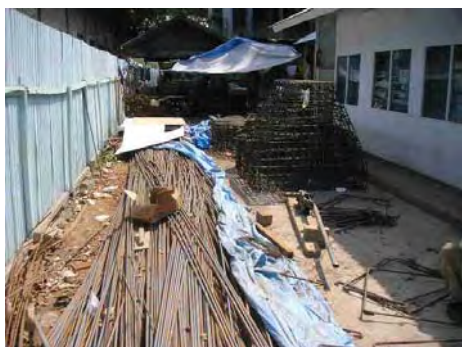
Construction materials processing factory (in front of field office)
