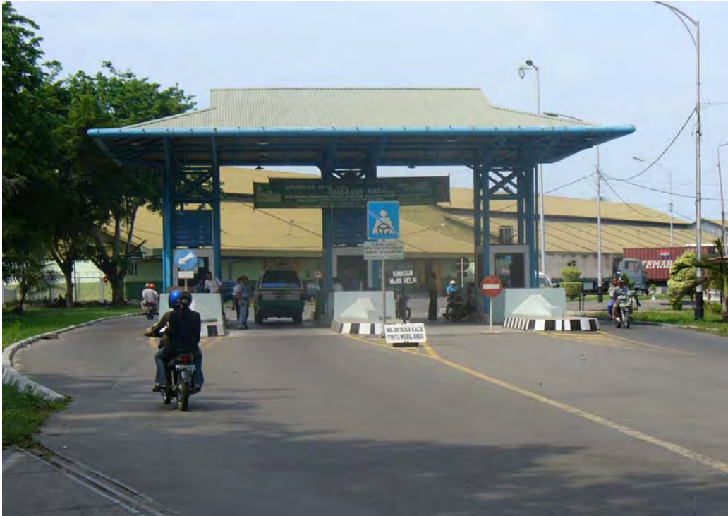
Access Control Gate (1)
