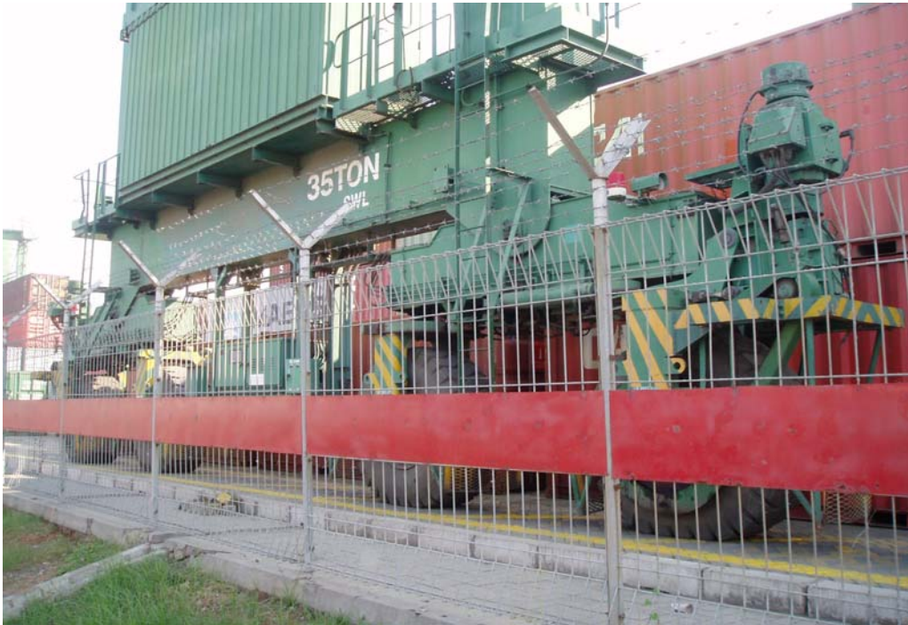
Restricted Area Boundary Fence with Top Guard
