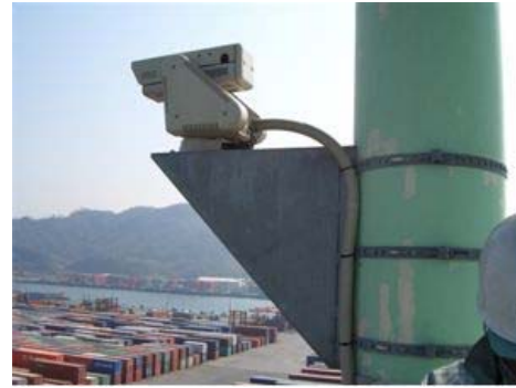
Above ↑ CCTV camera is on the lighting tower.
