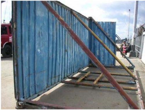
Mobile fence made of container (The inner bent part is a door.)
