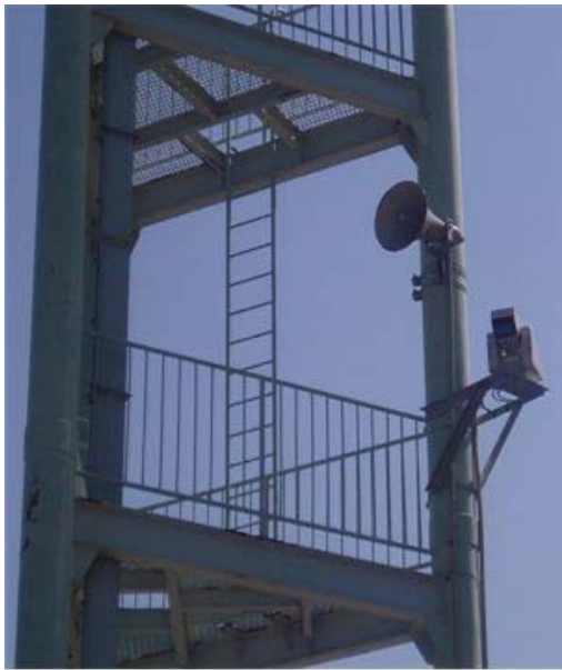
Above ↑ CCTV camera is on the lighting tower.
