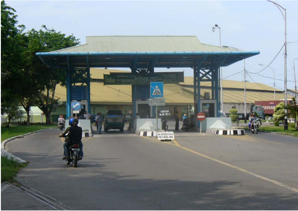
Access Control Gate (1)
