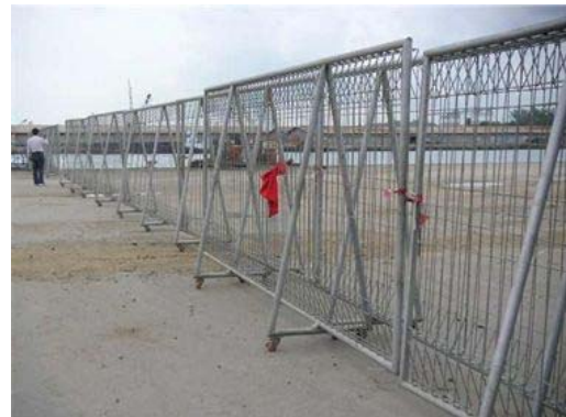
Mobile fences are in use as a partition between international vessel and domestic vessel.
