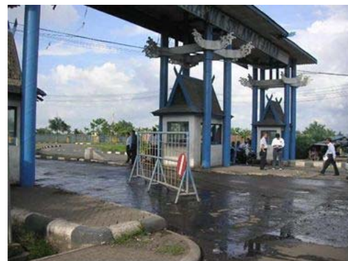
Mobile fence is used for the fence to prohibit vehicles to pass through.
