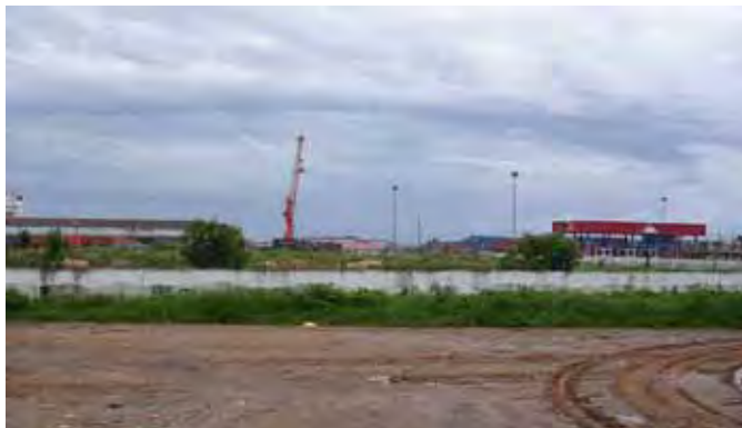
Concrete fence is provided along the port boundary. This area was reclaimed by excess soils from the construction site. Structure with a red roofing on the right side is the Gate no.3.
