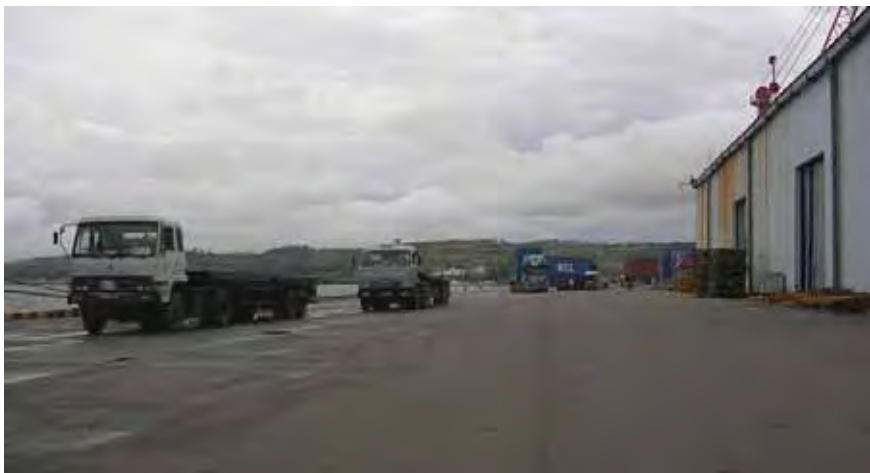
This is conjunction areas between the conventional wharf and container terminal.
