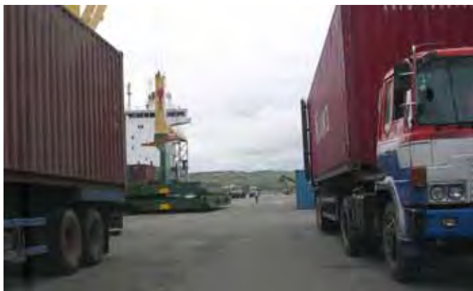
New container terminal is under construction to complete by 2007. After the completion, all containers will go through the Gate No.3.
