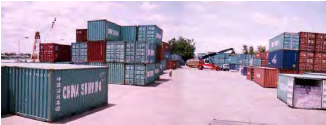
This is the import container stacking area which located at the end of the upstream side. The port length is about 500m but width is just 50 to 60m. PAP work hard to repair the and install the new fence to meet ISPS.
