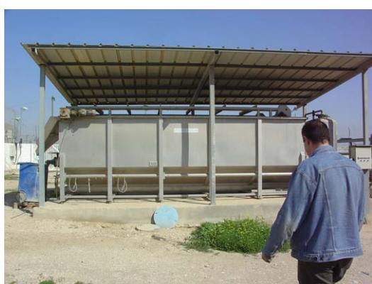
Pre-treatment plant for oil removal
