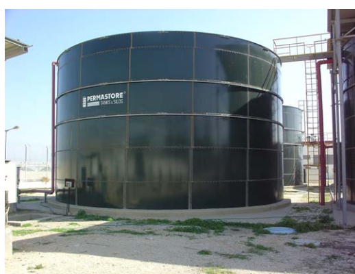
Aerobic Bioreactor (1 st tank, 24 hrs operation)
