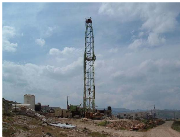
Construction of a New Well in Tammun
