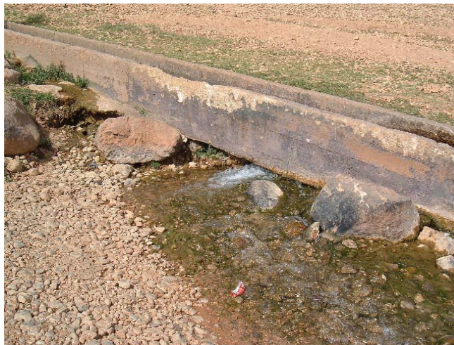
Water Leakage from a Channel (Al 'Auja Spring)
