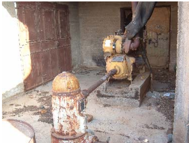
Non-operational Pumping Unit (Frush Beit Dajan)
