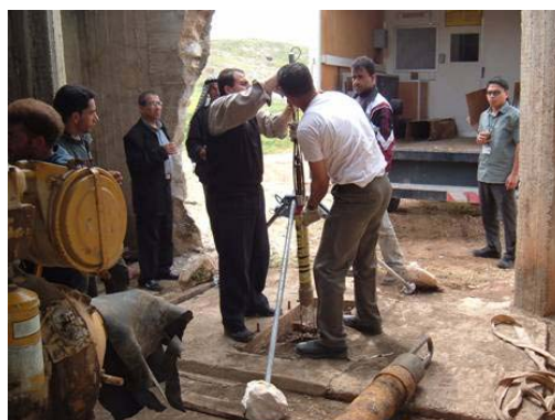
Setting of an Inspection Camera
