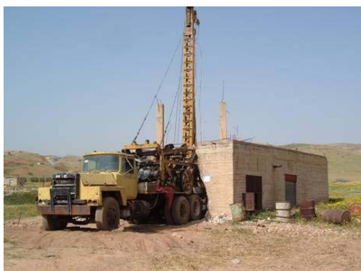
Rehabilitation of an Old Pump
