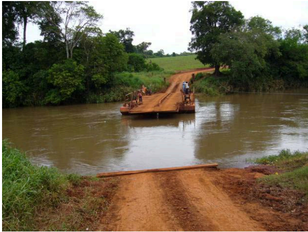
Pontoon Bridge crossing the Nacunday River
