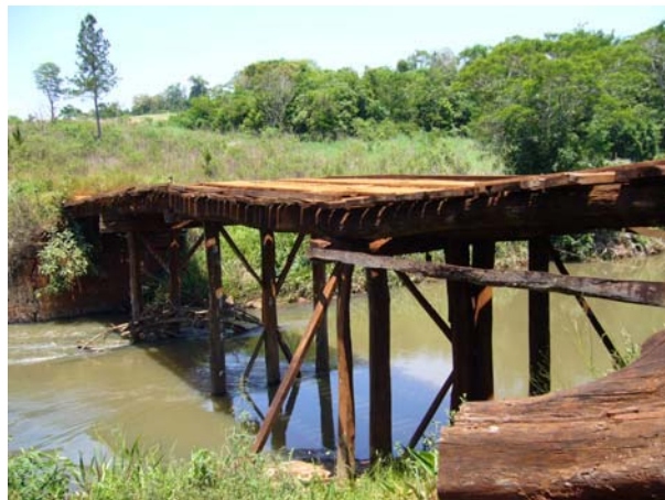
Timber Bridge crossing the Yacuy Guazu River
