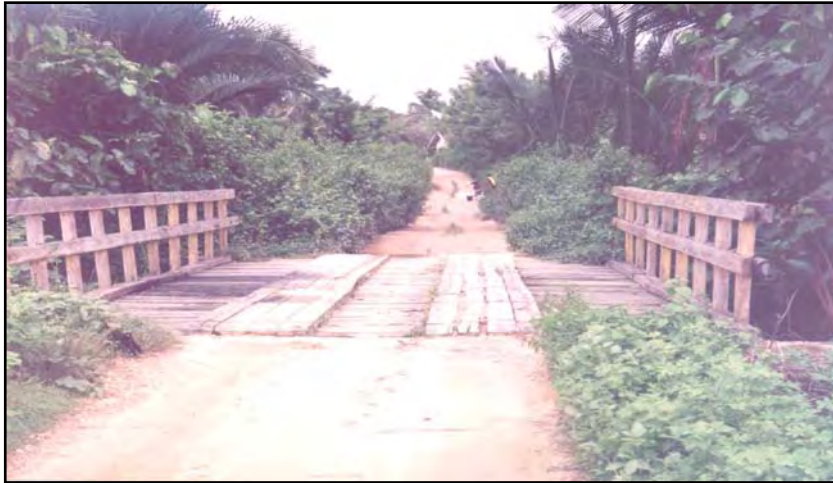
Road Bridge in Palangga village
