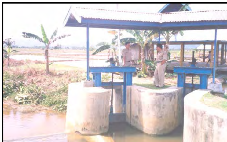
Check dam in Ranomeeto village
