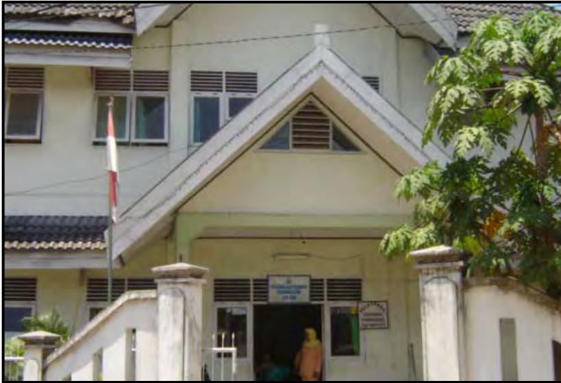
Community Health Center (Puskesmas), Bajeng, Gowa has been implemented PROAR
