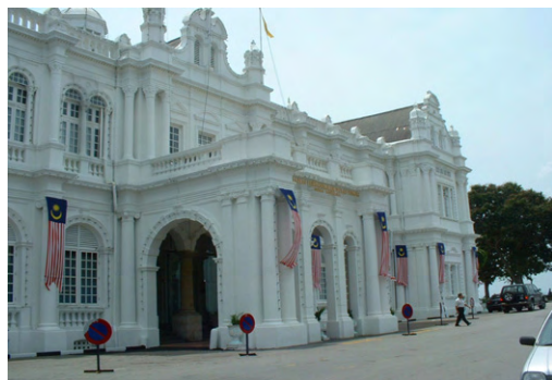
Plate 1: The MPPP Building at Padang Kota Lama, Penang
