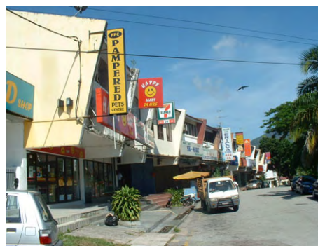
Houses and shops at Tanjung Bunga, MPPP
